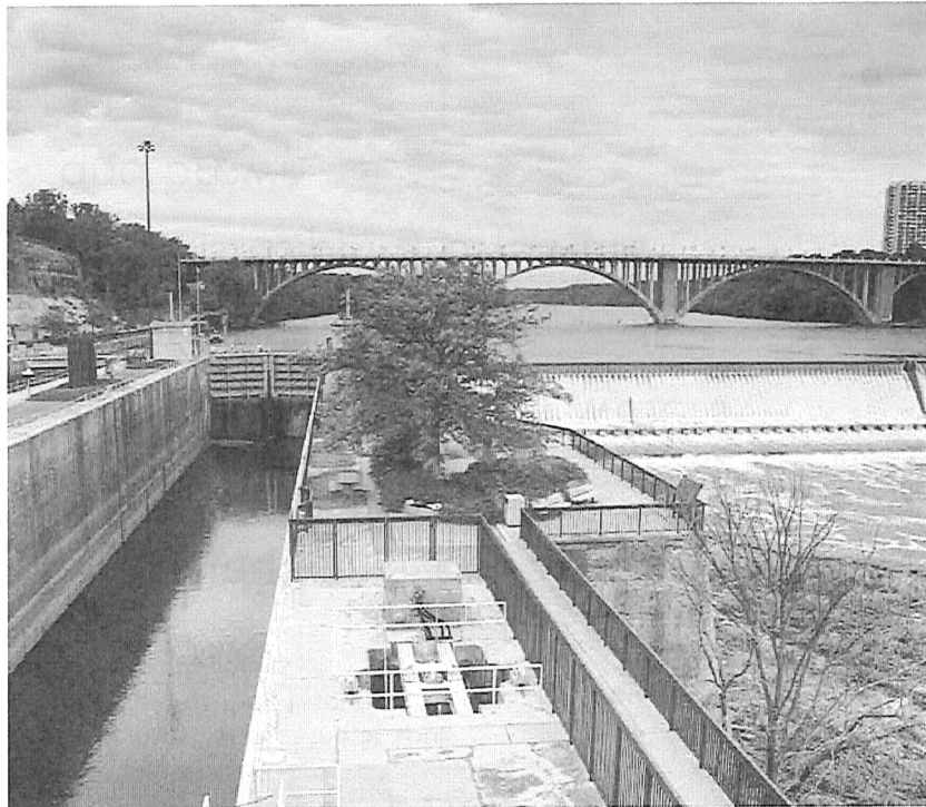
This lock (left) on the Upper Mississippi can raise or lower boats. Then they can pass around the dam (right) and continue along the river.
